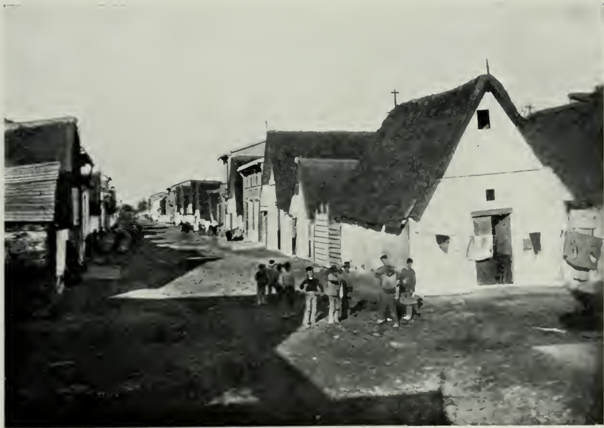
A ROAD IN CABAÑAL, ENVIRONS OF VALENCIA
